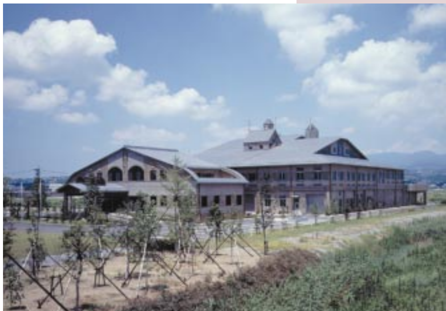
Night-soil treatment plant
