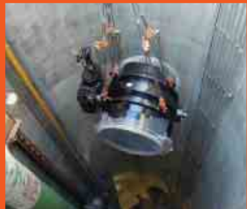
Metal-seated butterfly valve
