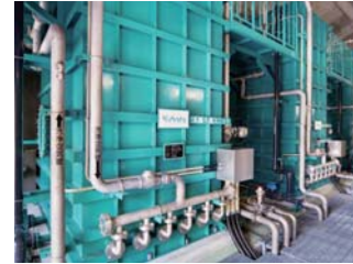
14 Ceramic film: used in the purification process for sources of water, including river water, to create clean drinking water.
