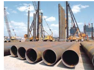
18 Spiral welded steel pipes: used in foundation construction, including for buildings and bridges in addition to harbor and river projects.
