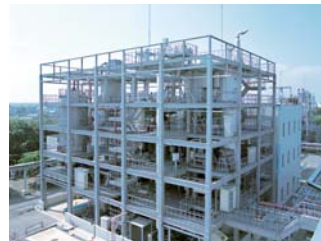
17 Sewage sludge incinerators: plants used to incinerate or melt sludge produced during sewage treatment
