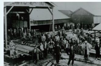
Kubota iron pipe shipping site around 1905
