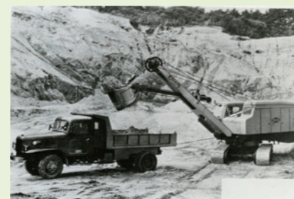
Mechanical power shovel performing loading (KB60 type)
