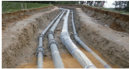
Ductile iron pipes: used in infrastructure, including water and sewage lines, and agricultural water facilities.
