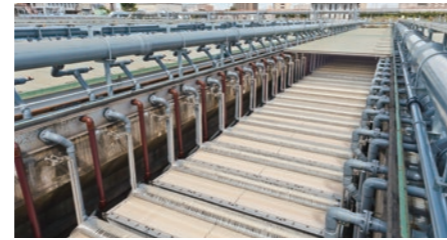
Submerged membranes: used to purify wastewater, including industrial and domestic sewage.
