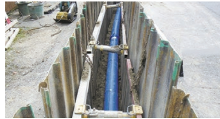
Plastic pipes: used in infrastructure, including water and sewage lines, and gas piping.
