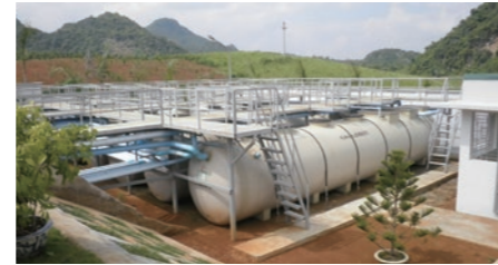
Wastewater treatment plants (Johkasou): used to treat wastewater in areas where there are no sewerage lines.
