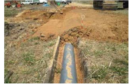
Pipes being buried in an open water channels
