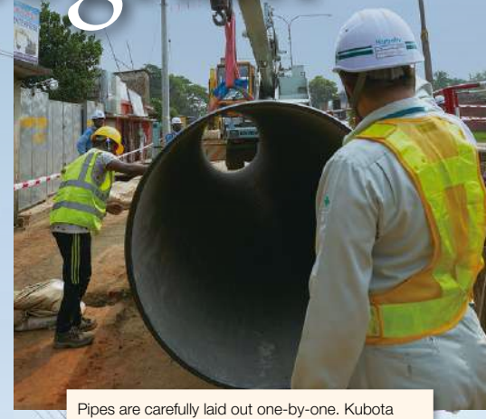
Pipes are carefully laid out one-by-one. Kubota also has unique knowhow in pipe connection.
