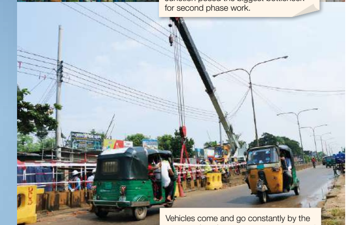
Vehicles come and go constantly by the construction site.
