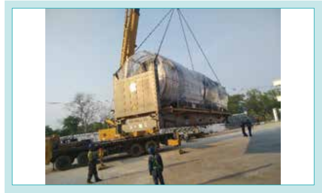
Fig. 6 Unloading at Site (Chemical Tank)
