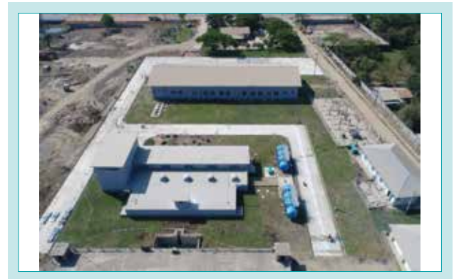
Fig. 10 Lagunbyin Pumping Station
