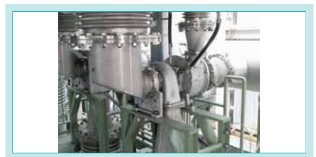
Fig. 5 Turbocharger
