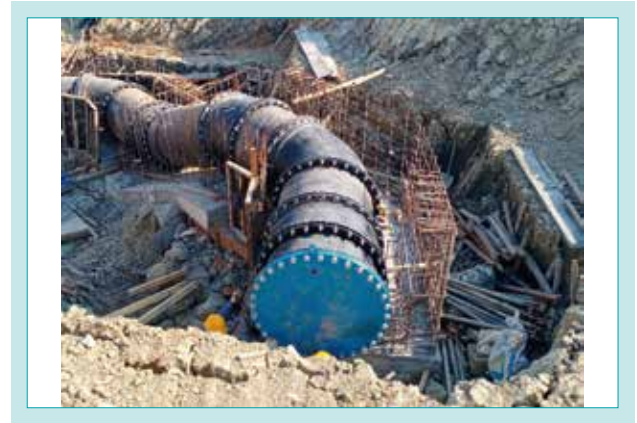
Fig. 9 Ductile Iron Pipe Installation (DN 1600 mm)
