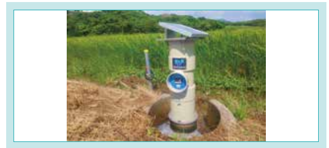
Fig. 5 Example of trial operation (Ishigaki City, Okinawa Prefecture)
