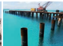
● Steel pipe piles
