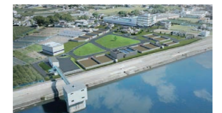
Artist's impression of the completed joint water treatment plant (Naruto City Enterprise Bureau)
