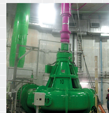
立軸渦巻斜流ポンプ (DS-VV型) Vertical volute type mixed flow pump (model: DS-VV) 口径: 300~3300mm 吐出量: 10~1500m 3 /min 全揚程: 3~20m 用途: 下水排水、汚水排水、雨水排水、農業用水等 Diameter: 300 - 3300 mm Discharge capacity: 10 - 1500 m 3 /min Total head: 3 - 20 m Use: Sewage drainage, polluted water drainage, rain water drainage, water for agricultural use, etc.
