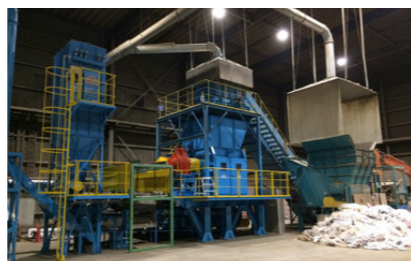
Plastic crushing and sorting facility
