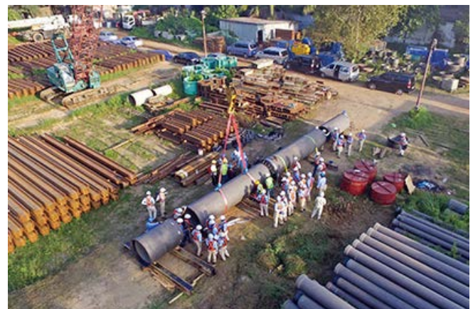
Instructing local engineers of the installation procedure
