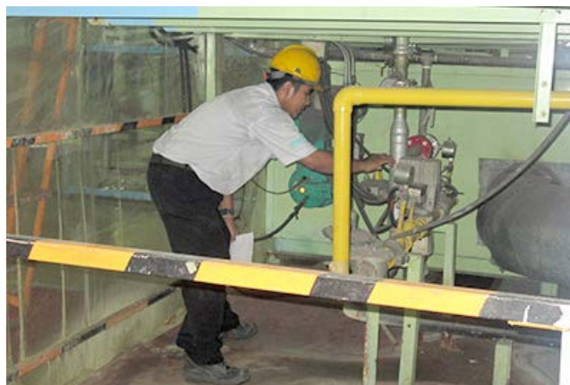
Emergency response drill simulating the leakage of gas P.T. Metec Semarang (Indonesia)
