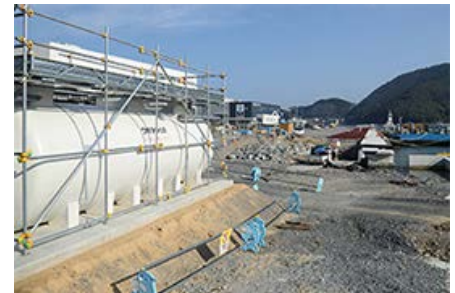
Wastewater treatment tanks (used to process wastewater from temporary housing and in regions with insufficient sewage lines)
