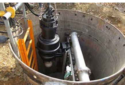
Manhole pumps (for pneumatic transportation of sewage)
