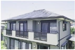
"Ecolony" solar power generating roofing tiles
