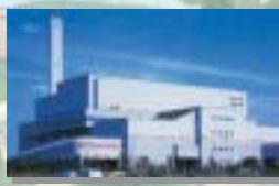
Municipal solid waste incineration plant with super generation
