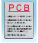
A label attached to the equipment containing PCB
