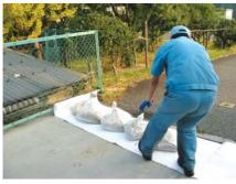
Use of oil mats and sand bags to prevent the Waste liquid which collects in a separation Any oil remaining in the final separation tank flow of waste liquid to gutters and/or other tank is sucked up by the vacuum vehicle locations
