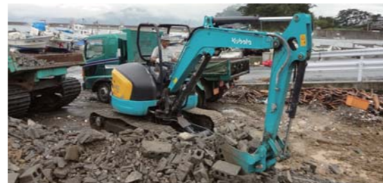
KUBOTA's construction machinery used actively to remove debris
