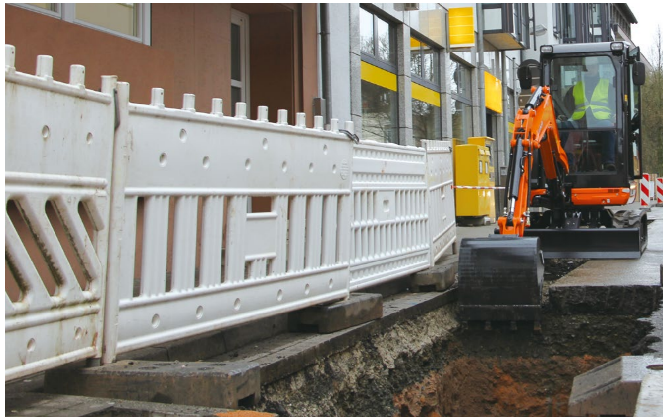
Mini excavators: used in civil engineering and other operations; especially useful in narrow work areas, such as city streets.
