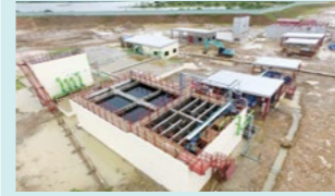
Water purification plant constructed in Thilawa Industrial Park
