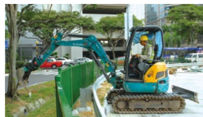
Mini excavator that can be used to develop urban infrastructure
