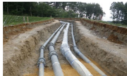
Ductile iron pipes: used in infrastructure, including water, sewage and agricultural water pipelines.
