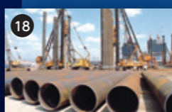
18 Spiral welded steel pipes: used in foundation construction, including for buildings and bridges in addition to harbor and river projects.
