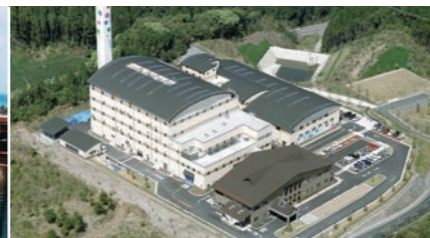
● Waste incinerator plants / ash and melting furnace plants used to incinerate and reduce the volume of municipal waste, as well as to contribute to decarbonization of society by generating electricity utilizing high-temperature waste heat.
