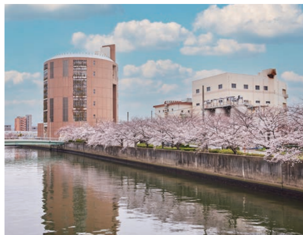
Nakahama Sewage Treatment Plant in Osaka
