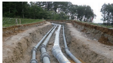
● Ductile iron pipes used in infrastructure, including water, sewage and agricultural water pipelines.
