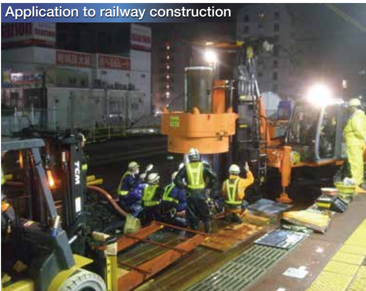
*Example of night time construction during railway tracks closing
