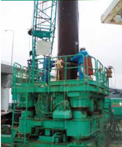
Rotation pressing-in pile Method
