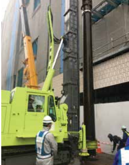
Screwed pile Method
