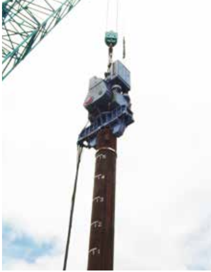
Vibro-hammer Method
