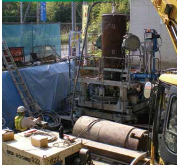
Hydraulic rotation Center Bored pile Method
