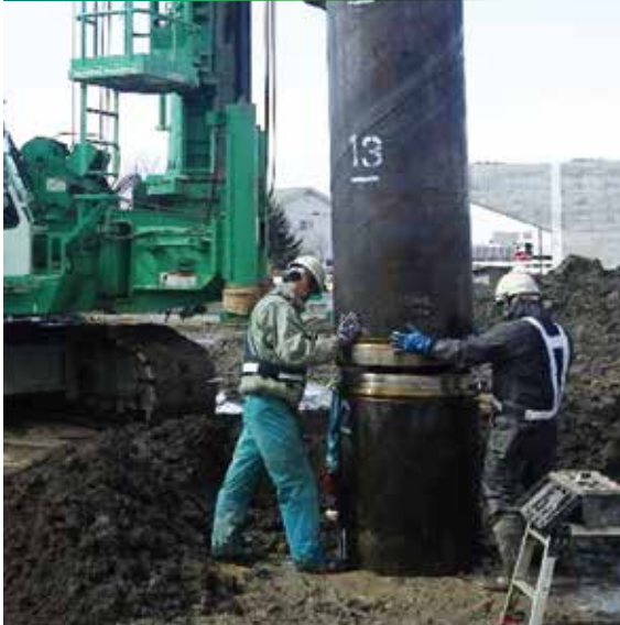
Center Bored pile Method
