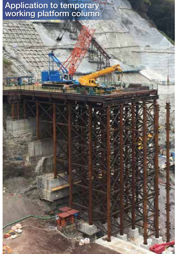
*Example of application to platform columns
