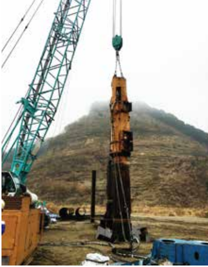
Pile driving Method
