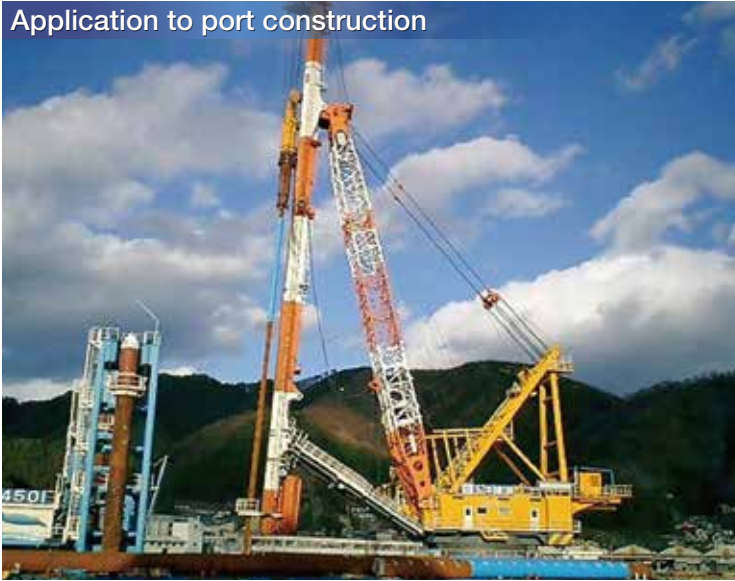
*Example using a pile driving barge
