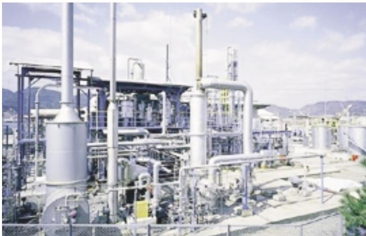
Waste Plastics Liquefaction Plant
