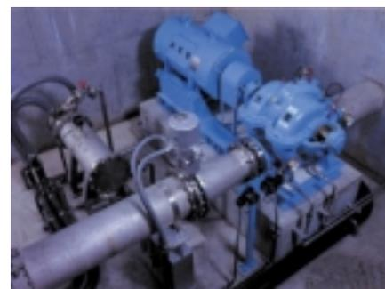
Pump with reverse rotation impeller
