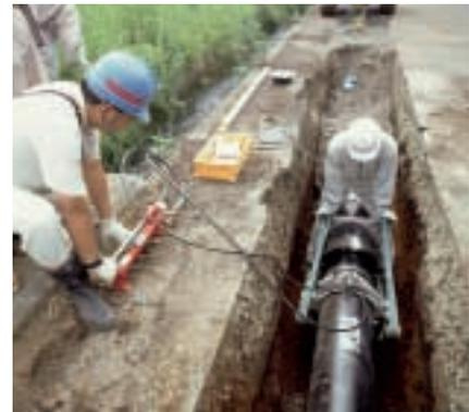
NS quake-resistant joint parts of ductile iron pipes
