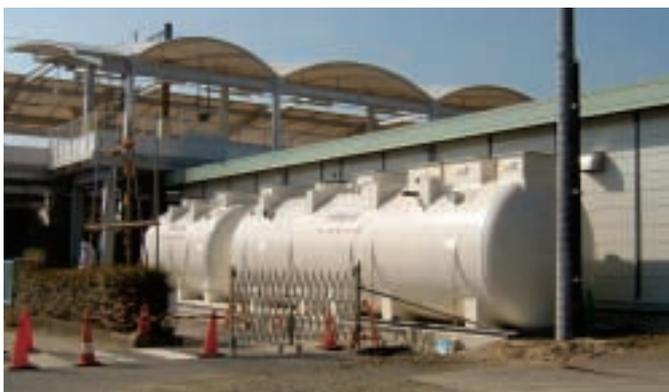
The Wastewater treatment tank with advanced membrane process installed at the Banpaku-yakusa station
