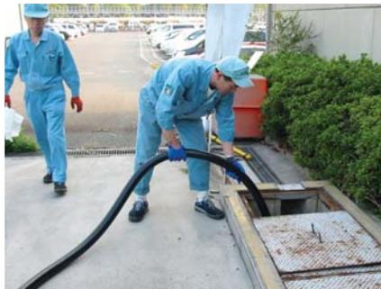
Waste liquid which collects in a separation tank is sucked up by the vacuum vehicle
