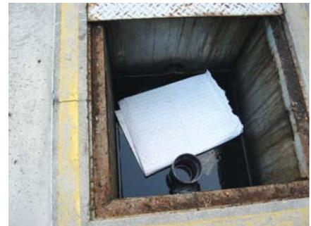
Any oil remaining in the final separation tank is absorbed with an oil mat
