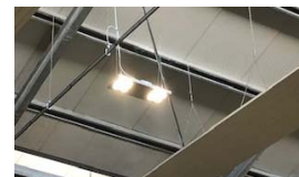
LED lighting installation
