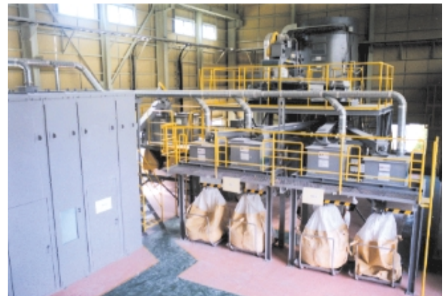
The pilot plant of crashing waste F.R.P. bathtubs
