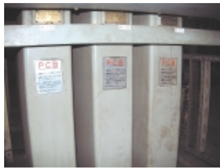
A label attached to the equipment containing PCB
