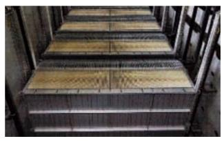
Sewage treatment equipment in the Fukusaki Water Purification Center, Fukusaki-cho, Hyogo Submerged membranes units installed in reaction chambers
