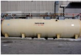
Joukaso installed in a hotel in Saga Prefecture K-HC-R2: 436 people, 88 m³/day (flow control tank + concentrated sludge tank)
