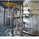
Three gun burner (gas gun) units are installed in the incinerator.
