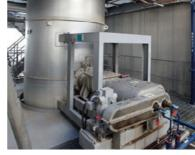
Dewatered sludge (in the form of dewatered cakes) is fed here. 2.5 tons of dewatered sludge per hour is inserted into the continuous type
