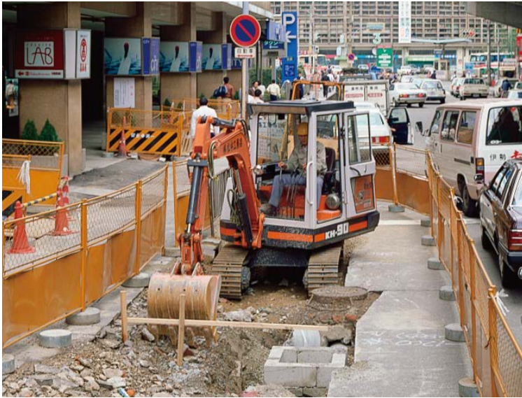
Mini excavator KH90 at a narrow construction site near Osaka Stadium
