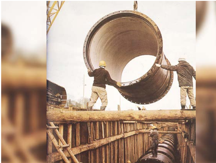
Laying the extra-large-diameter 2200mm ductile iron pipes
