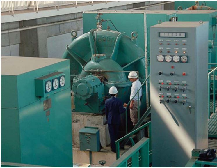
The then nation's top class 3,100kW double-suction volute pump delivered to Shizuoka City Department of Municipal Enterprise
