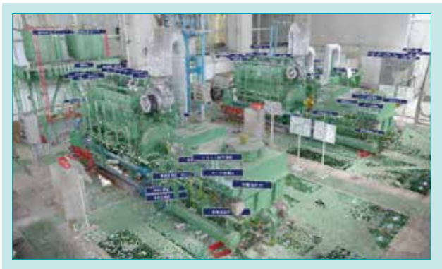
Fig. 4 Flag Inspection Points Overlaid on 3D Point Cloud Data
