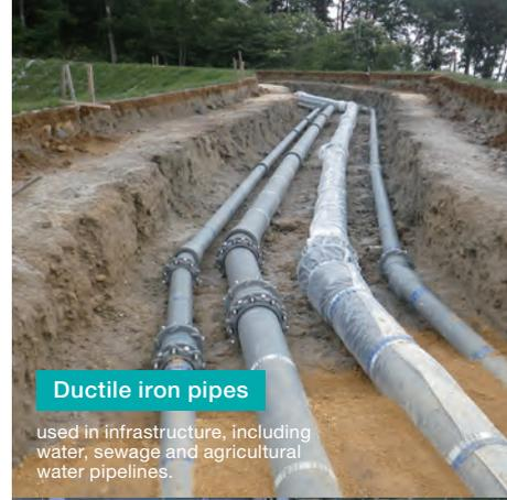
**Ductile iron pipes**
