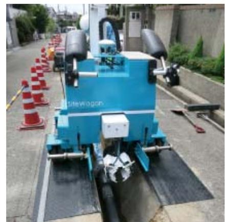
Pipe laying using side wagon
