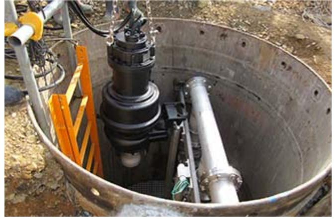
Manhole pumps (for pneumatic transportation of sewage)
