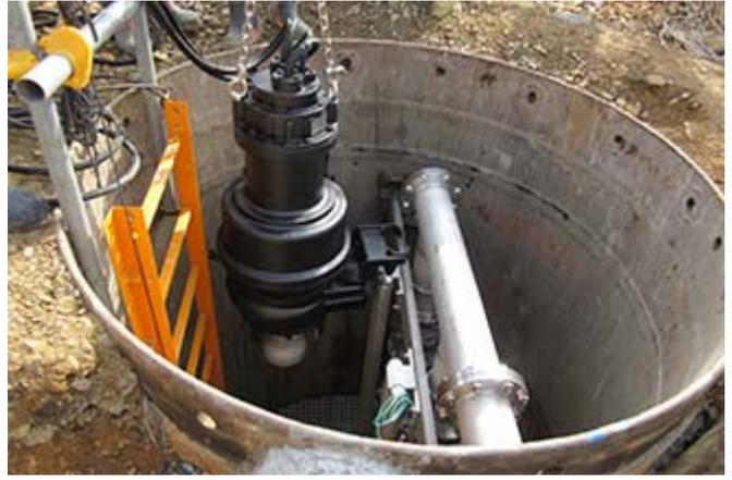
Manhole pumps (for pneumatic transportation of sewage)
