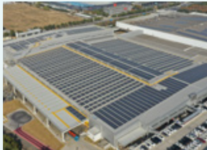
Solar panels installed
