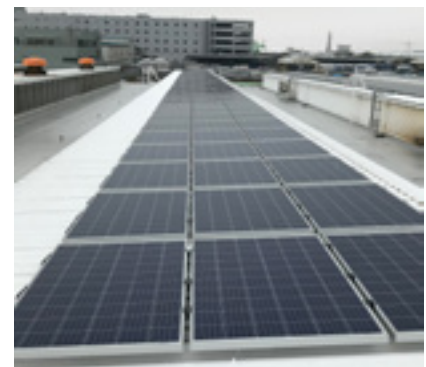
Installation of solar power generation system Kubota Sakai Rinkai Plant
