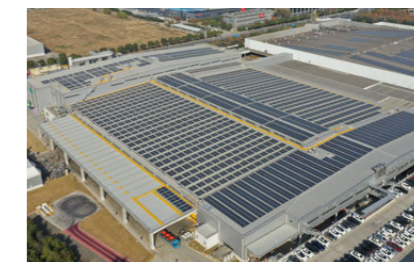
Solar power generation system installed on the rooftop of a plant in China
