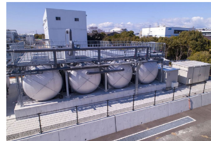
At the Kubota Sakai Rinkai Plant (Japan), we expanded our installation of submerged-type FRP johkasou , decentralized wastewater treatment plants. These are able to handle high-level treatment of household wastewater and can process up to 110 m 3 of wastewater per day. Furthermore, as a BCP measure, we have raised the concrete foundations of the wastewater treatment facility. We introduced a water management solution using IoT, "KSIS," to realize proper management of plant wastewater.
