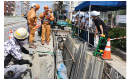
Installation of earthquake-resistant water pipes
