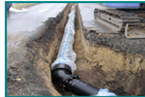
Construction of earthquake-resistant pipes in area of distress
