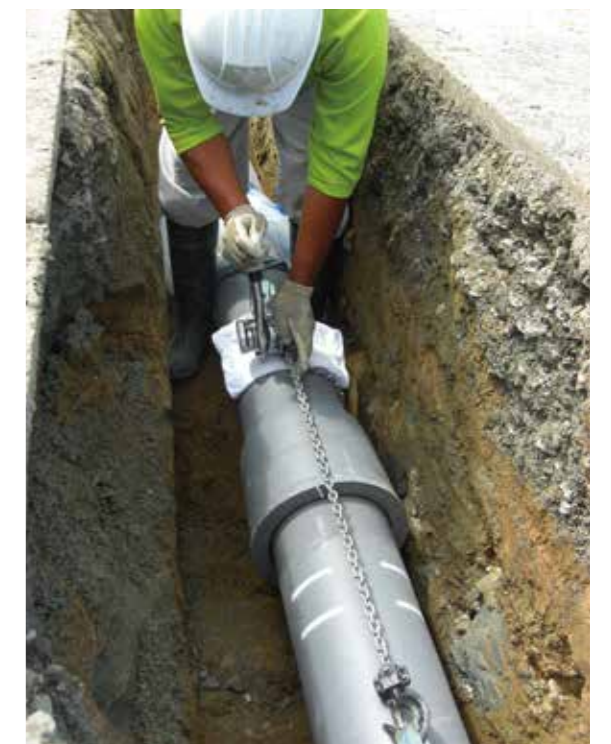
Joining work of push-on joint (GX-type)
