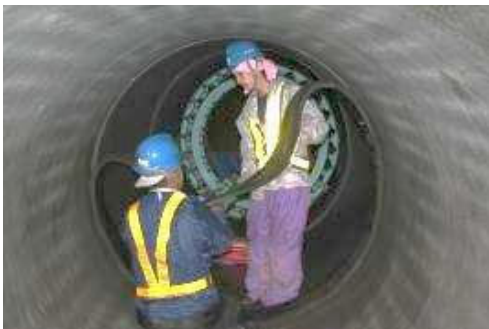
Pict.13 Rubber Ring in the center of a joint
