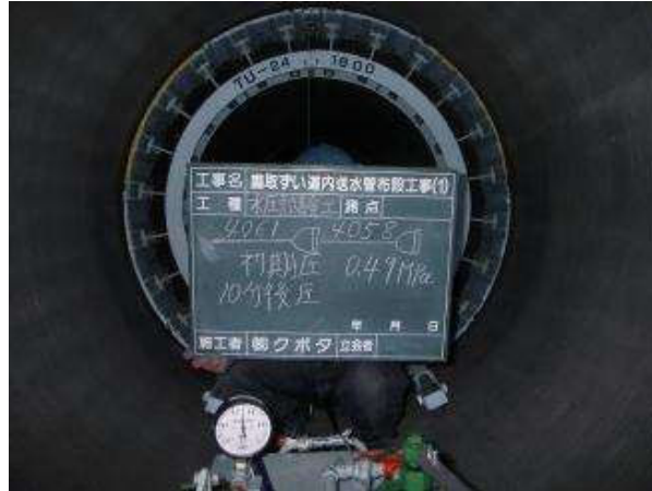
Pict.16 Hydraulic pressure test
