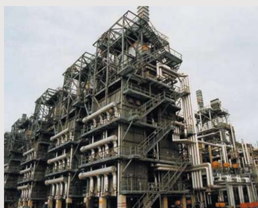
Cracking Furnace in Nova Chemicals
