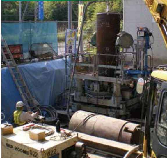
Hydraulic rotation Center Bored pile Method
