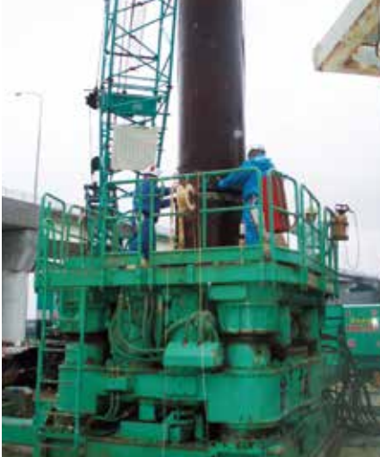
Rotation pressing-in pile Method
