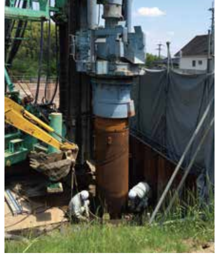
Composit pile Method of Steel pipe pile and soil cement
