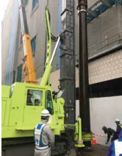
Screwed pile Method
