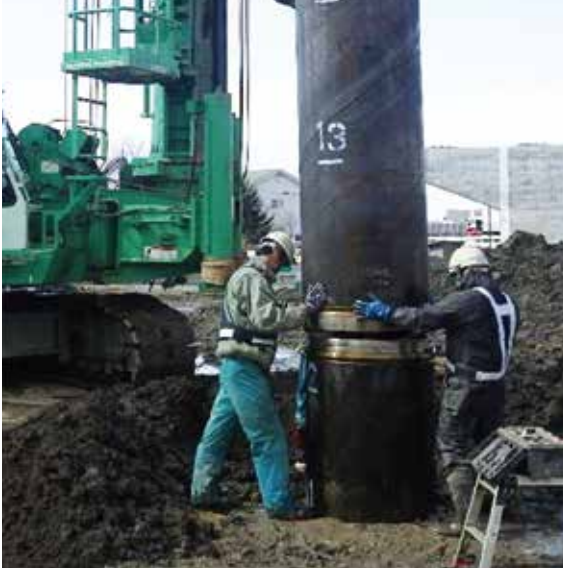
Center Bored pile Method
