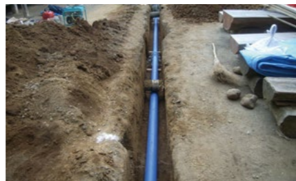
Plastic pipes: used in infrastructure, including water and sewage lines, and gas piping.
