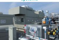
Sakai Plant: Utilizing the waste heat generated at the time of in-house power generation and reducing the consumption of steam boiler fuel
