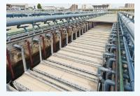
Kubota's submerged membrane units—which decontaminate sewage and industrial wastewater—help solve wastewater treatment issues worldwide.
