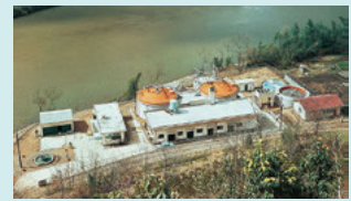
Night soil treatment plant in Miyoshi, Hiroshima, the first project after the Division was formed
