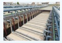
Kubota's submerged membrane units—which decontaminate sewage and industrial wastewater—help solve wastewater treatment issues worldwide.
