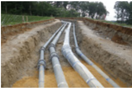
Ductile iron pipes: used in infrastructure, including water, sewage and agricultural water pipelines.
