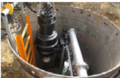
Manhole pumps (for pneumatic transportation of sewage)
